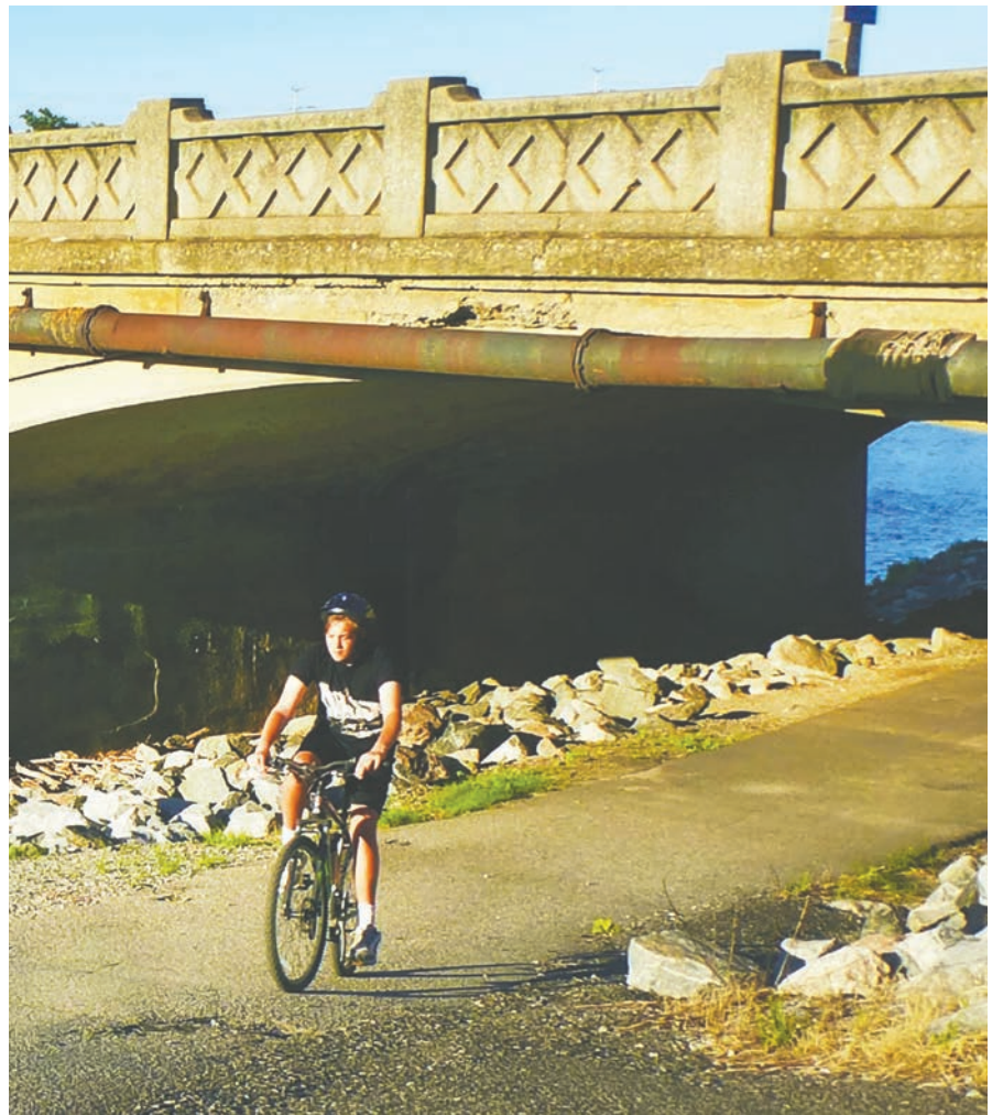
Along the south flood wall.
