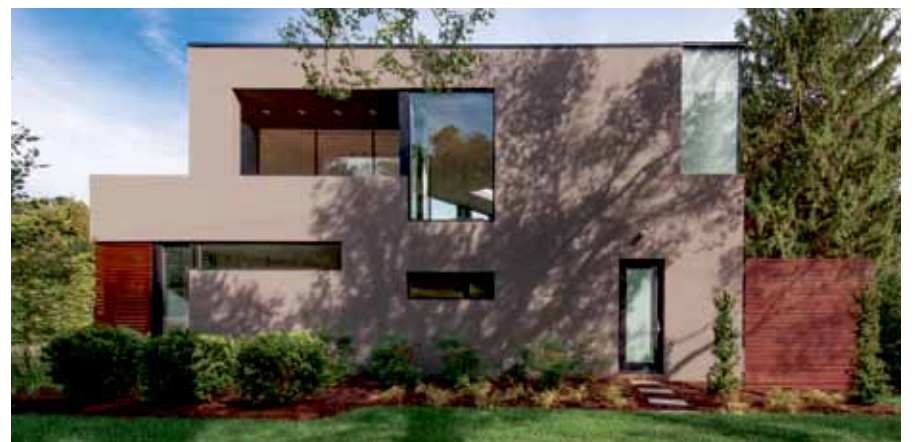
Top: Round Hill Farm Pavilions and Landscape in Orange, Virginia. Designed by Spatial Affairs Bureau, Charlottesville, Virginia. The design team included Peter Culley, Stacey Farinholt, Andrew Montgomery and James Hill.
